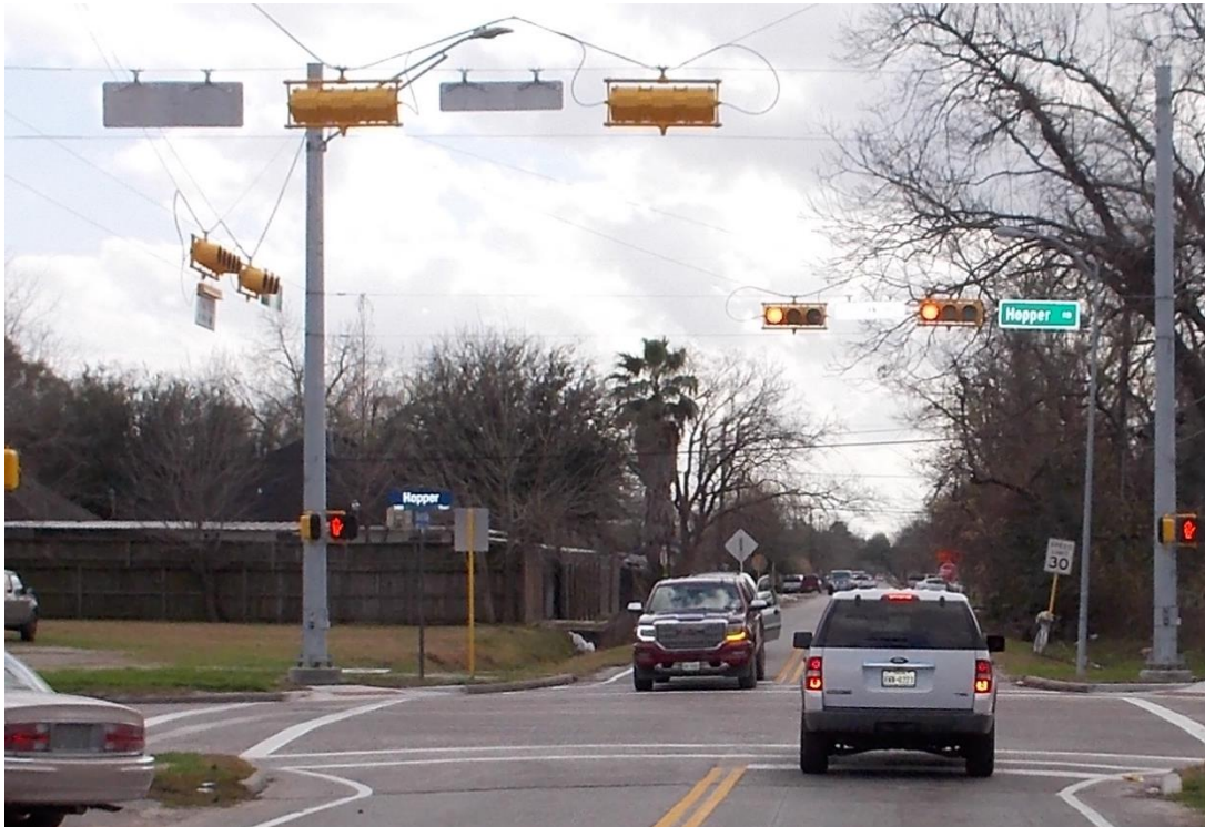
New traffic signal at Hopper Road and Seven Mile Lane in East Aldine is now operational.
