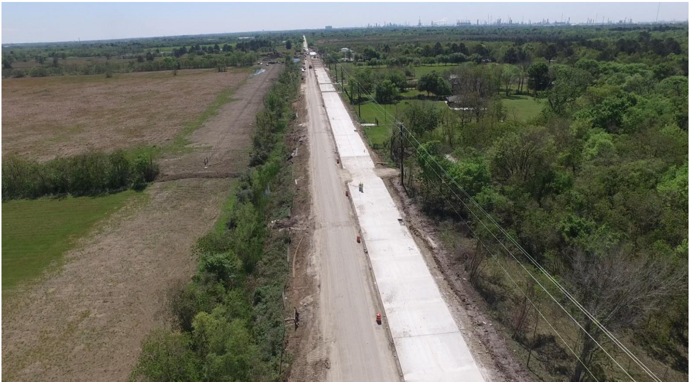
Construction along John Martin Road during the roadway shutdown.
